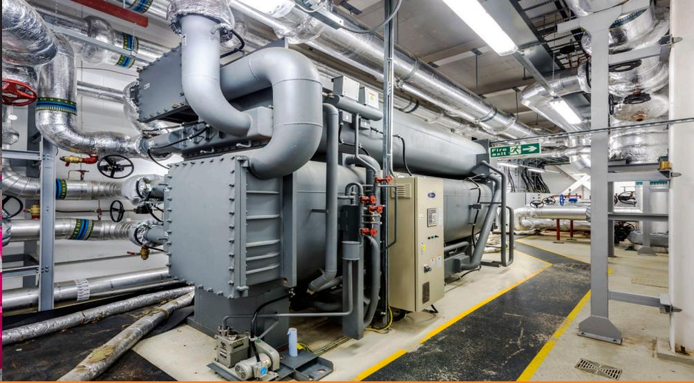
*The scheme not only makes use of the waste heat generated, but also allows the CHP engine to run more hours and closer to full capacity, which makes it more efficient and commercially beneficial. The electricity generated from the CHP also feeds the plant in the cooling pod which has an overall cooling capacity in excess of the peak load and can fully meet the anticipated peak cooling of the buildings it serves.*
