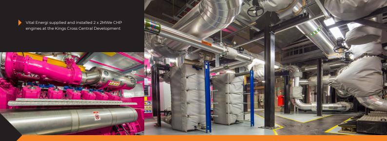
One of the challenges facing Vital Energi was designing an energy centre in a building which was largely uncompleted. Initially the energy centre and car park levels were completed, but another 14 stories were later added to the building. As these were not completed during the energy centre installation we needed to create free-standing chimneys which needed to be 55m high to adhere to the clean air act.
