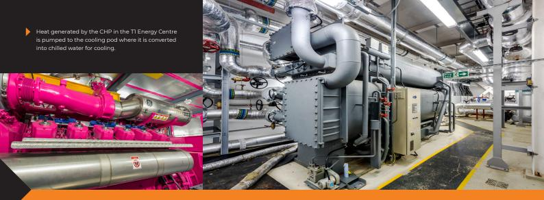
The scheme not only makes use of the waste heat generated, but also allows the CHP engine to run more hours and closer to full capacity, which makes it more efficient and commercially beneficial. The electricity generated from the CHP also feeds the plant in the cooling pod which has an overall cooling capacity in excess of the peak load and can fully meet the anticipated peak cooling of the buildings it serves.
